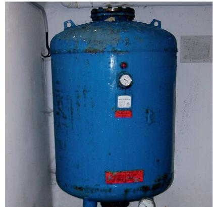
Fig. 2: Corrosion and rust
