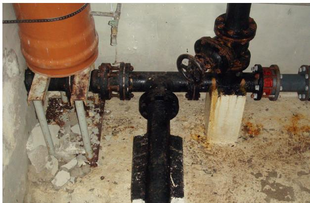
Fig. 3 : Moisture penetration damage
