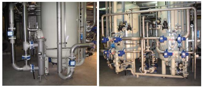
Condensate polishing line with resin trap
