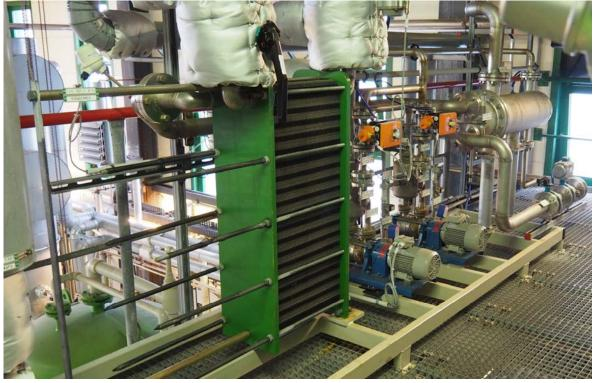
Rack with vapour condenser, vacuum pumps and additional preheater for feed water (from right to left) Referenz rwt014
