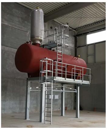
Degasification after erection
