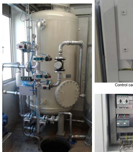
Filter vessel with automatic front piping
