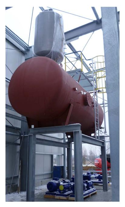
Customer: Procedure: Capacity: Year of realisation: Specialities: Power plant operator Thermal degasification 45 t/h 2013 Degasification plant with measurement and safety instrumentation, vapour condenser, substructure and access platform
