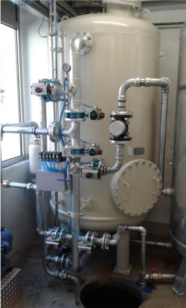
Filter vessel with automatic front piping
